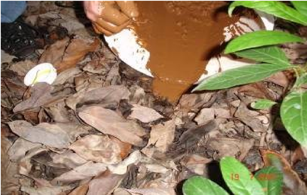
Figure 2. Preparing the slurry mixture – Soil collected during drilling is mixed with water to form a slurry. Carefully pour the mixture to avoid air pockets
