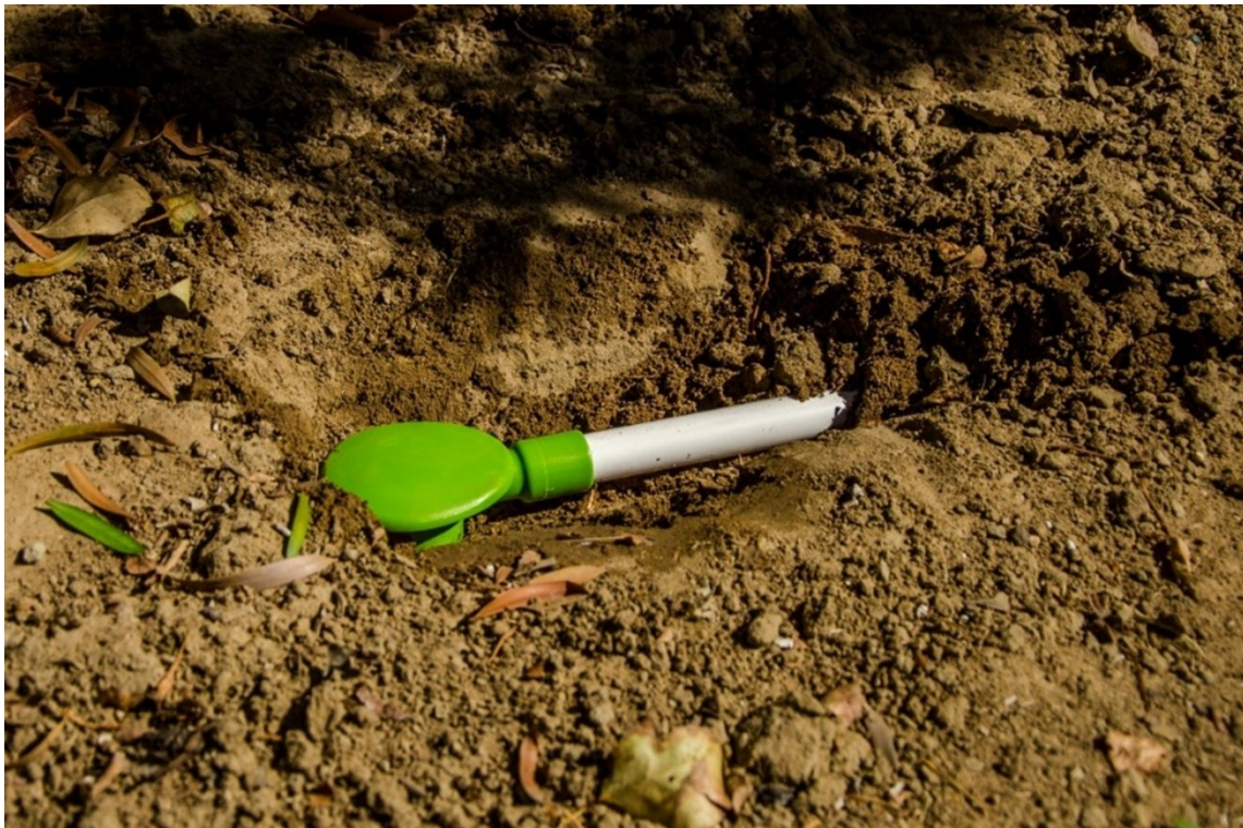
Figure 4. Concealing the probe cable – Make use of plastic conduit to conceal and protect the probe cable. Cover up the trench with loose soil and lightly compact.
